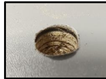
2 – DRILLING INTO SLAB
