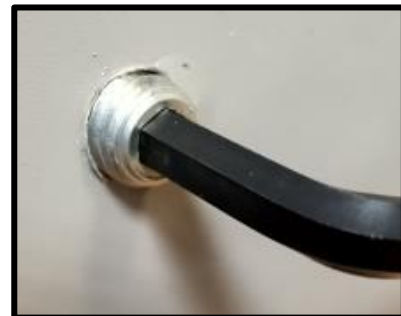
3 – INSERTING BRACKET INTO SLAB
